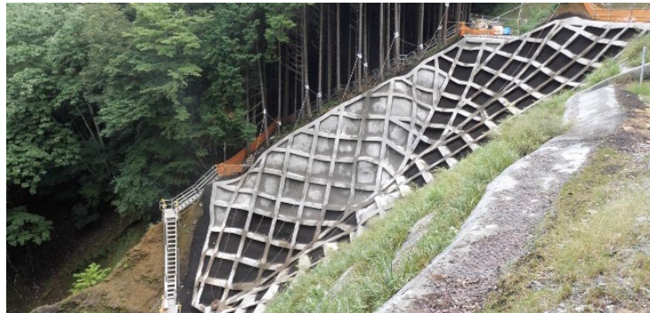
Slope site where survey was conducted. Taking pictures of uneven slopes was difficult with conventional autonomous operation, but is now possible leveraging the know-how we have cultivated at the Company.
