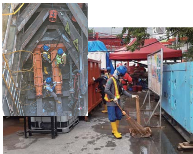
■マカッサル市北西域下水幹線工事 Cement Soil Mixing Demonstration Work Development of Makassar City Northwest Zone
