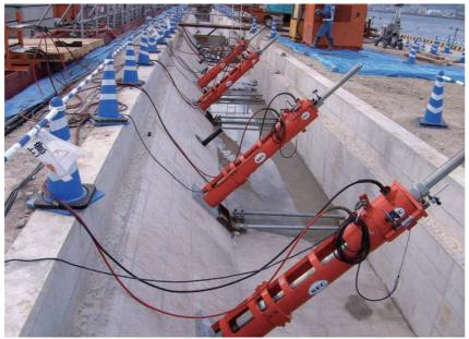
Simultaneous tightening of multiple anchors
