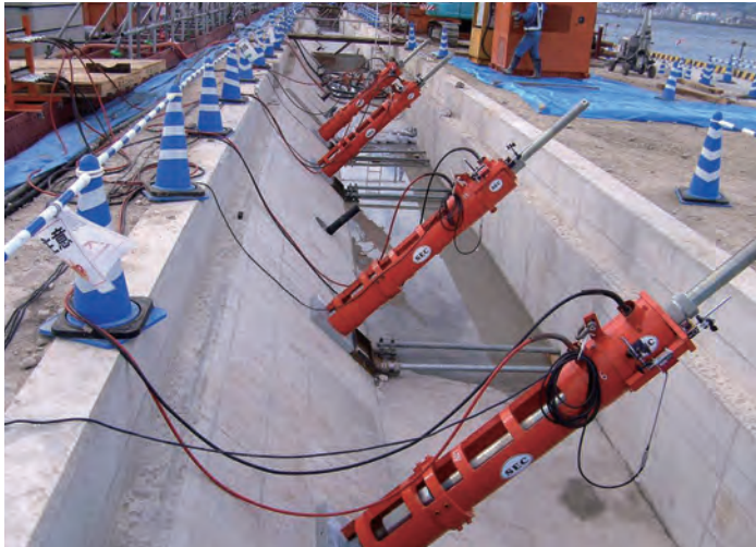
Simultaneous tightening of multiple anchors
