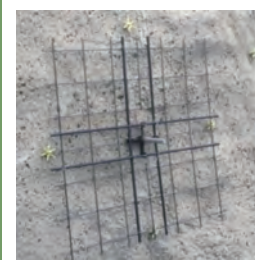
Installation of reinforcing material
