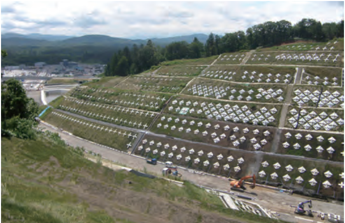
Ground anchors + Pressure receiving plates
