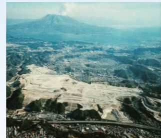
Site preparation for land readjustment project in Ishiki, Kagoshima-shi, 1997
