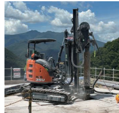
Construction of electricity tower foundation (SC-TEP Drill No. 2)
