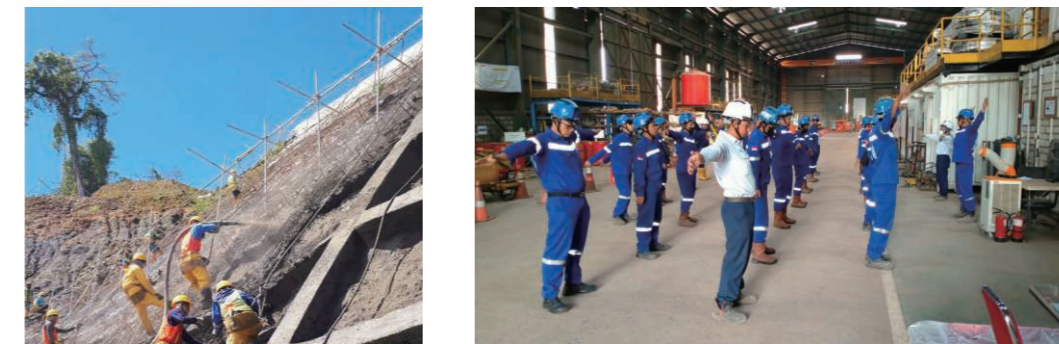
Works in charge: Slope frame work
