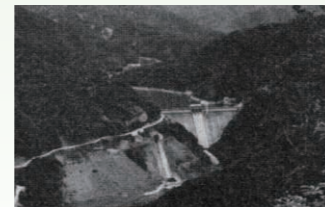
The Saso River Dam construction project, the beginning of our advance into central Japan Constructed between 1956 and 1958
