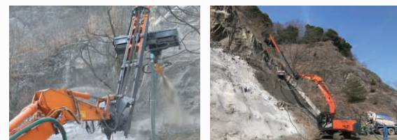
Spraying on rock slopes
