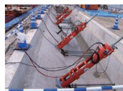
Simultaneous tensioning of multiple anchors
