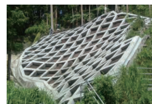
Sprayed slope frames
