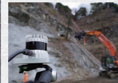
Slope spraying with Slope Savior. Simultaneously monitor spraying thickness using LiDAR.
