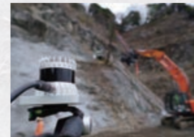
Slope spraying with Slope Saver. Simultaneously monitor spraying thickness using LiDAR.
