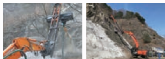
Spraying on rock slopes
