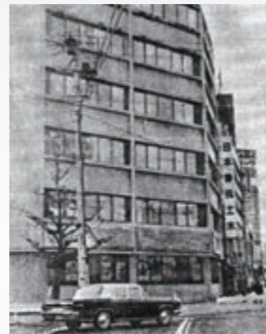
Ginza headquarters building
