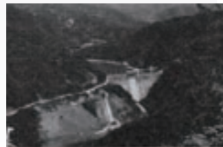
The Saso River Dam construction project, the beginning of our advance into central Japan. Constructed between 1956 and 1958
