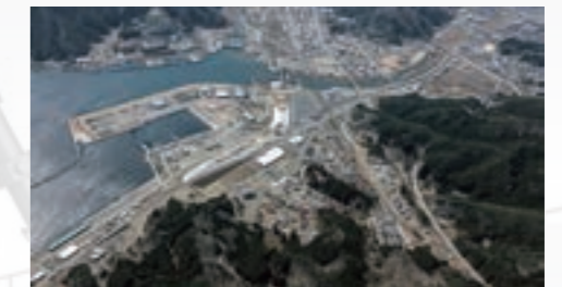
Ando area, Otsuchi-cho reconstruction work 2019
