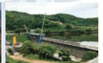
Senbon Dam foundation reinforcement work 2020
