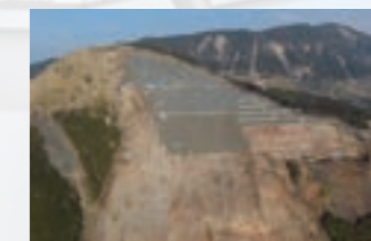
Aso Ohashi area slope protection work (Aso-gun, Kumamoto) 2017
