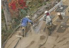
Sand from the left-side nozzle and polyester continuous fiber from the right-side nozzle are injected by jet water to form continuous
