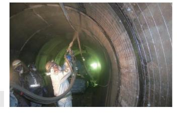
Pumping distance: 1,000 m (with a hose extension) Design strength: 18 N/mm<sup>2</sup> or more
