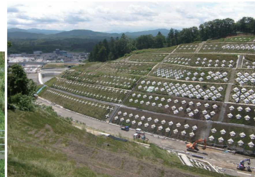
Ground anchors + Pressure receiving plates
