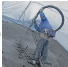
Spraying of fiber-reinforced mortar
