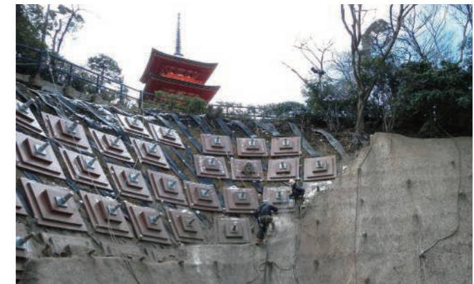
Slope under the Koyasu-no-tou, a National Important Cultural Property
