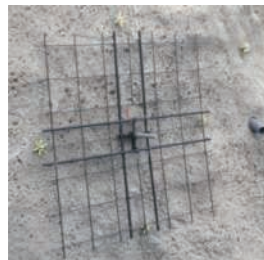
Installation of reinforcing material
