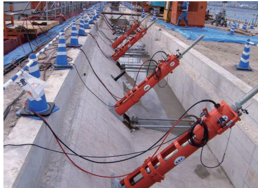
Simultaneous tightening of multiple anchors
