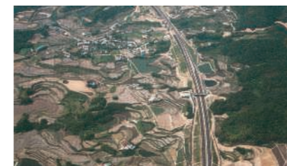
National Route No. 28 Yasuhira Work of the Honshu-Shikoku Bridge Authority (Awaji Island, Hyogo Prefecture)
