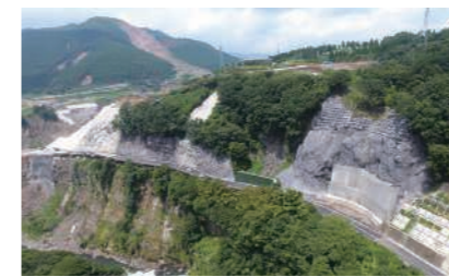
Kumamoto Earthquakes Disaster Restoration Work
