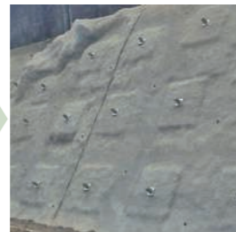
Completion of work
