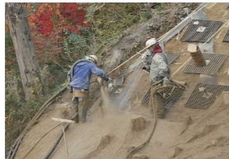
Sand from the left-side nozzle and polyester continuous fiber from the right-side nozzle are injected by jet water to form continuous fiber-reinforced soil.
