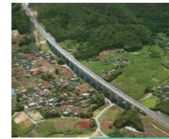
Ogitsu Work of Joban Expressway, Japan Highway Public Corp. (Ibaraki Prefecture)
