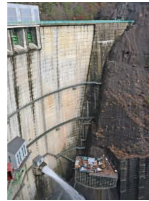
Construction of Kawamata Dam (2017)
