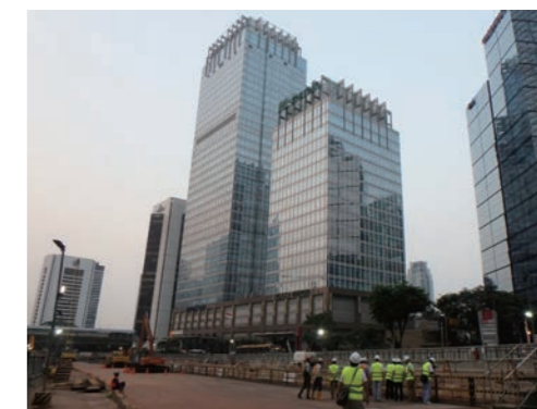
Construction of Jakarta Mass Rapid Transit Project
