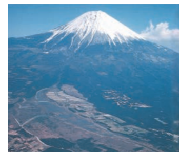
Mt. Fuji Osawa Collapse Countermeasure Works of the Ministry of Construction (Shizuoka Prefecture)
