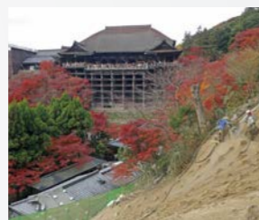
During the work
