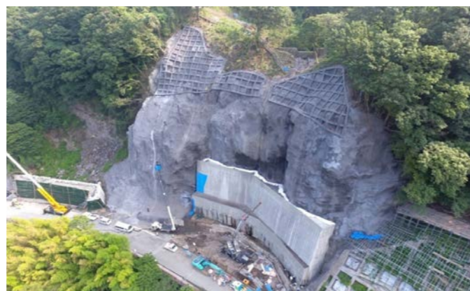
During the work
