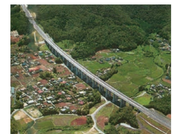
Ogitsu Work of Joban Expressway, Japan Highway Public Corp. (Ibaraki Prefecture)
