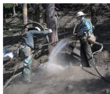
Sand from the left-side nozzle and polyester continuous fiber from the right-side nozzle are injected by jet water to form continuous fiber-reinforced soil.
