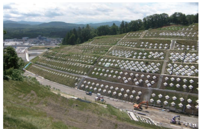
Ground anchors + Pressure receiving plates
