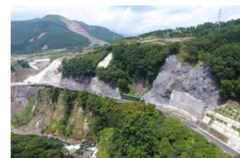
Kumamoto Earthquakes Disaster Restoration Work
