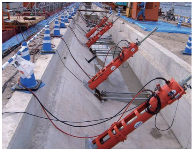
Simultaneous tightening of multiple anchors
