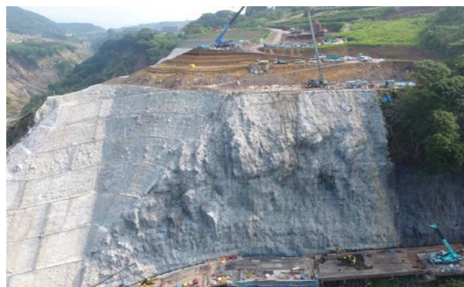
During the work
