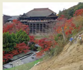
During the work
