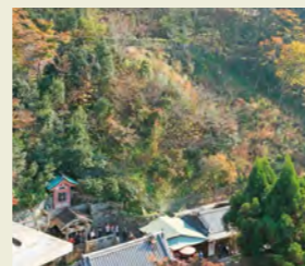
One year after the work completion
