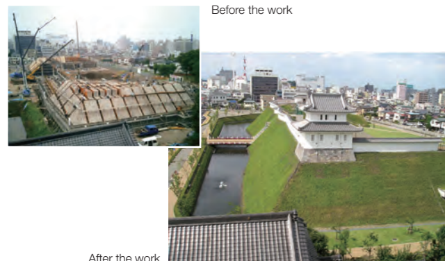
After the work
