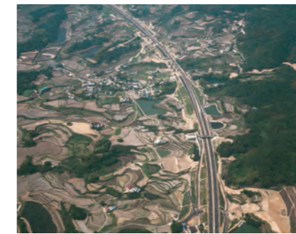
National Route No. 28 Yasuhira Work of the Honshu-Shikoku Bridge Authority (Awaji Island, Hyogo Prefecture)
