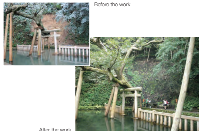
After the work
