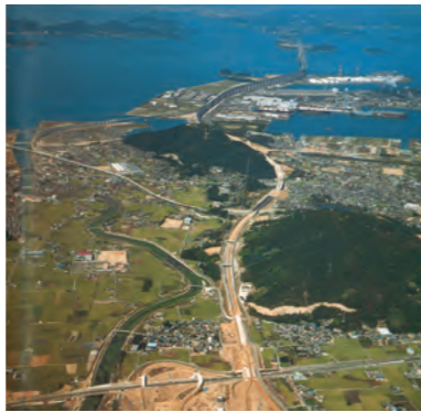
National Route No. 30 Mukaiyama-minami Work of the Honshu-Shikoku Bridge Authority (Kagawa Prefecture)
