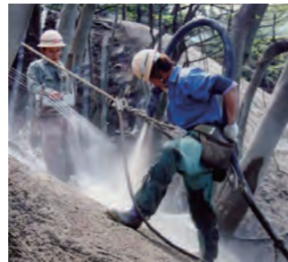
Sand from the right-side nozzle and polyester continuous fiber from the left-side nozzle are injected by jet water to form continuous fiber-reinforced soil.
