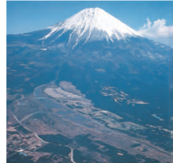
Mt. Fuji Osawa Collapse Countermeasure Works of the Ministry of Construction (Shizuoka Prefecture)
