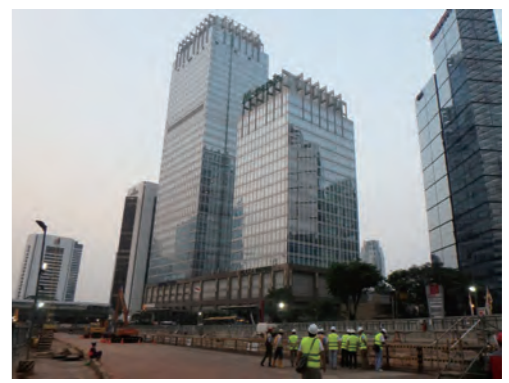
Construction of Jakarta Mass Rapid Transit Project
