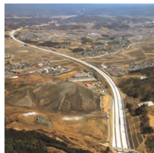
Sakai Section of Joban Expressway, Japan Highway Public Corp. (Fukushima-Pref.)
