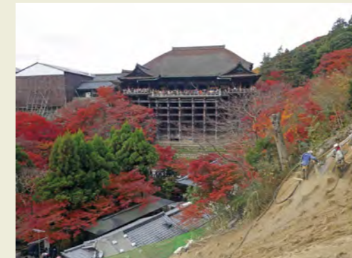
During the work
