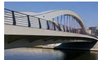
Shin-Toyo Bridge in fiscal 2007
