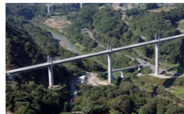
Fudo Ohashi Bridge (former Yamba Dam Lake No. 2 Bridge) in fiscal 2010
