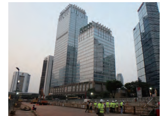
Construction of Jakarta Mass Rapid Transit Project
