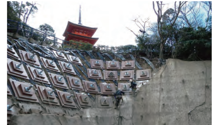
Slope under the Koyasu-no-tou, a National Important Cultural Property
