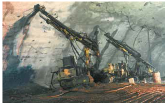
PS anchor and grouting at underground power plant
