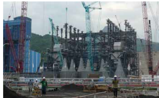
Soil improvement for thermal power plant foundation
