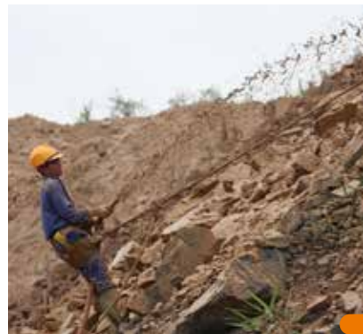
Spraying of Seeds and Foundation Soils
