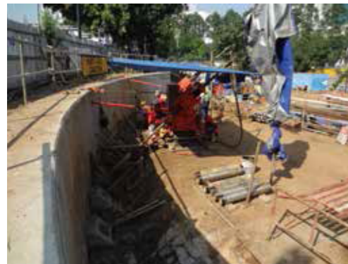
Earth retaining temporary anchor for the station building
