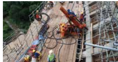
Ground Anchor Work in Progress
