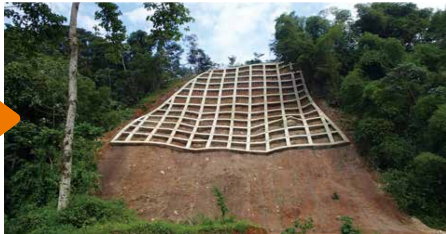
Construction Work Completed
