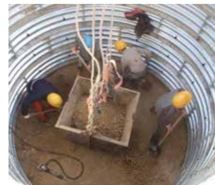
Slope Stability Project Well, Drilling & Installation of Drainage Pipe, Piles (SV)
