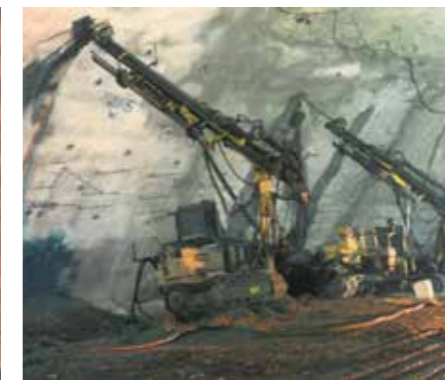
Hydroelectric Power Station Project PS-Anchor, Dam Grouting
